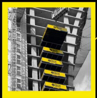
Able to be stacked vertically, SuperDecks are retractable and can be used as a drawer-like system.
