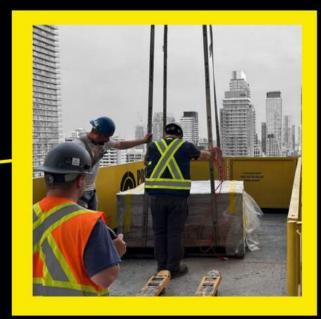
Installed vertically in as little as 15 minutes, using a two prop method or a bolt down method.
